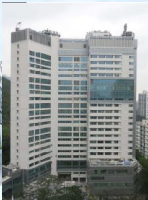
The Converted SSQ (Block T)
