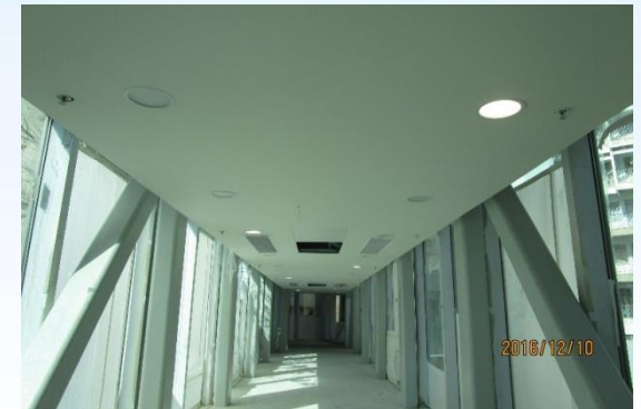
E&M installation at Link Bridge
