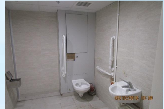
Accessible toilet installation at L17
