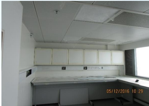
Lab furniture installation at L18
