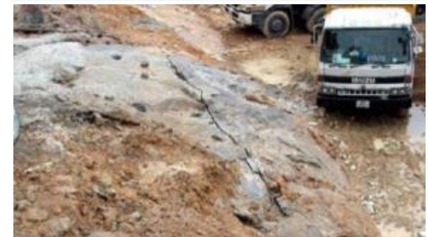
Chemical reactions will induce cracks in the rock mass a few hours later (i.e., during night time)
