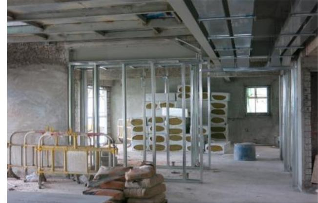
Installation of Drywall at L16
