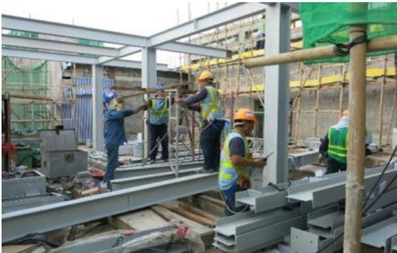
Installation of Building Maintenance Unit (BMU) steel frame at L23 roof floor
