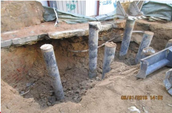
Excavation works for pile caps for the construction of link bridge
