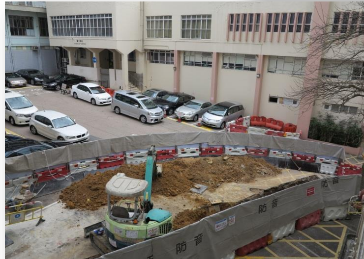
Underground utility diversion works
