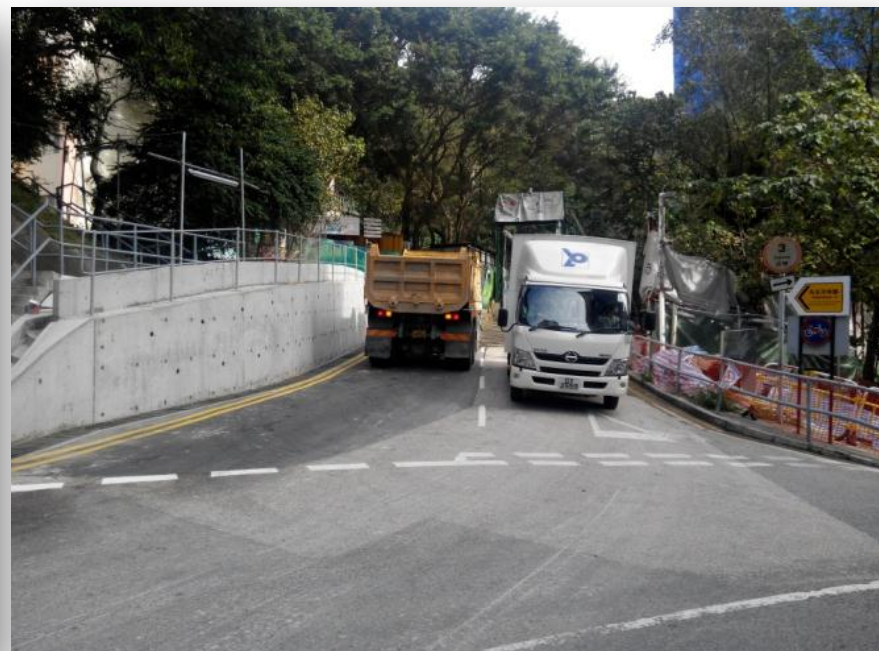
AFTER Road Widening Works
