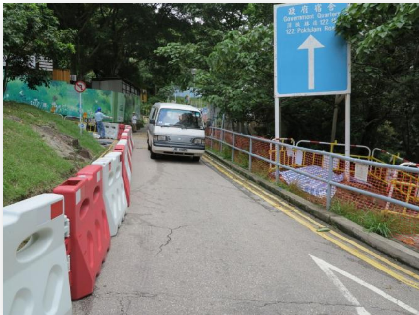
BEFORE Road Widening Works
