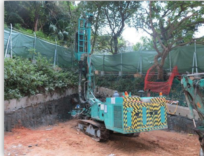
Diversion of drainage pipes
