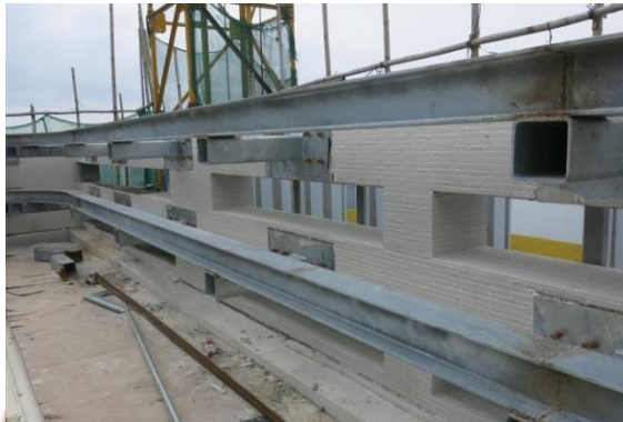
Installation of Building Maintenance Unit (BMU) at L24
