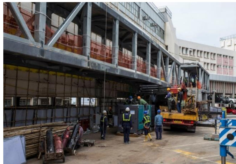
Steel truss fabrication works for the construction of link bridge
