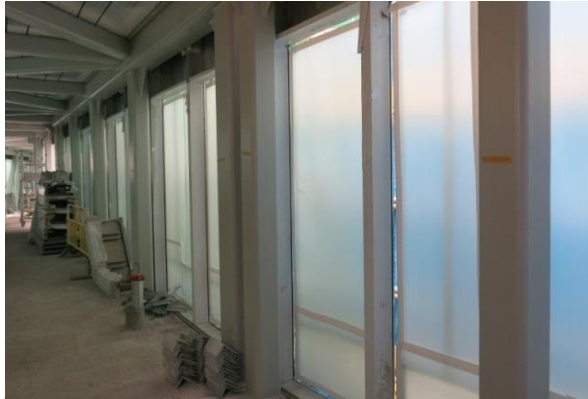
Installation of cladding and glazing at link bridge
