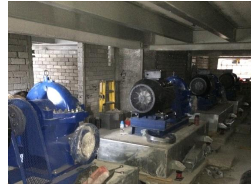
Chilled water pumps were delivered to site
