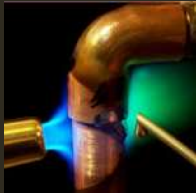
Welding pipes
