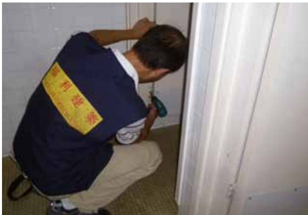
Staff of TMS(BW) repaired door hinge
